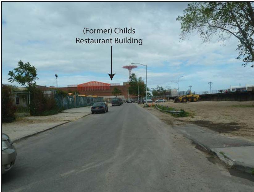
3. View east along Highland View Avenue from West 23rd Street, with the (Former) Childs Restaurant Building in the background.
