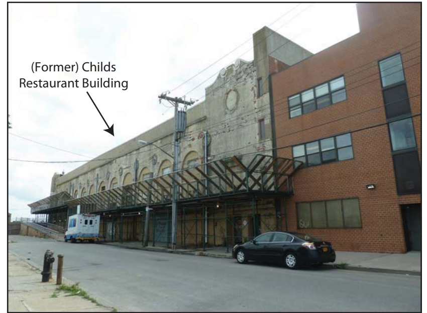
6. View southwest across West 21st Street of the (Former) Childs Restaurant Building and adjacent NYC Medicaid office building.
